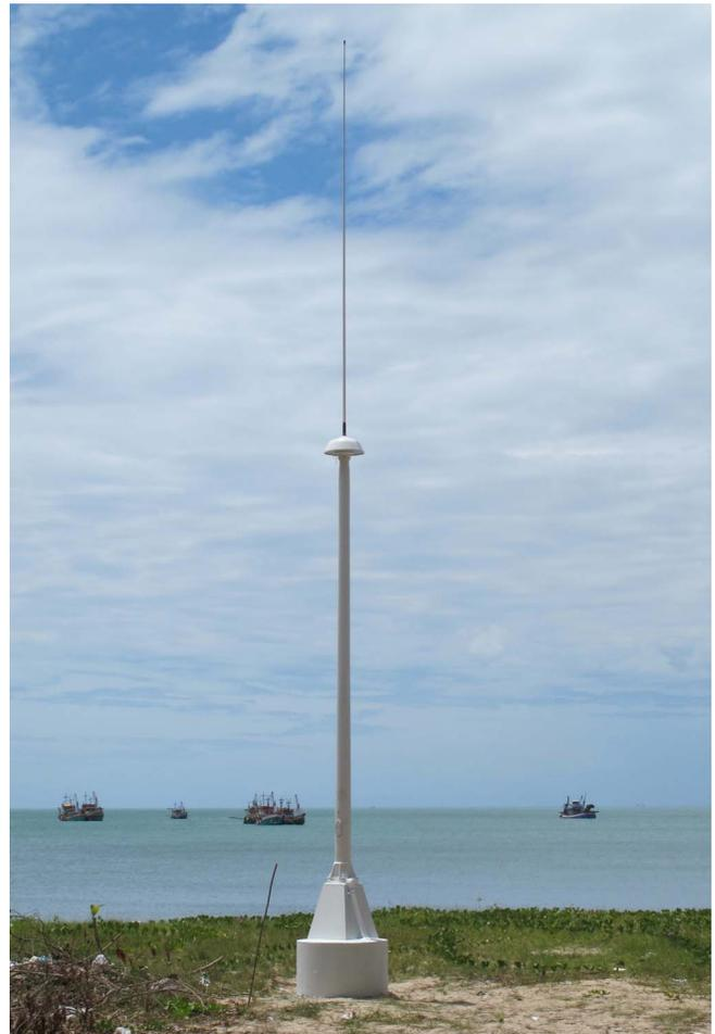
Fig. 1. SeaSonde compact cross-loop antenna installed at coast.
